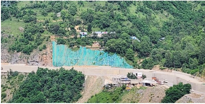
Slope Protection work under construction
