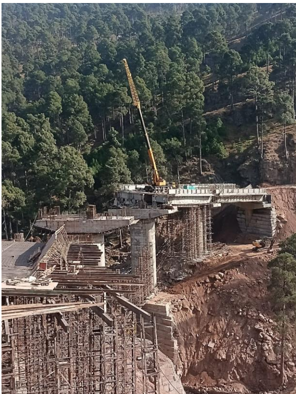
MJB 2 Under Construction
