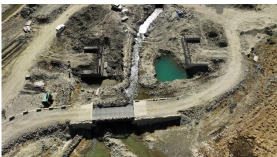
MNB 30 m span under construction
