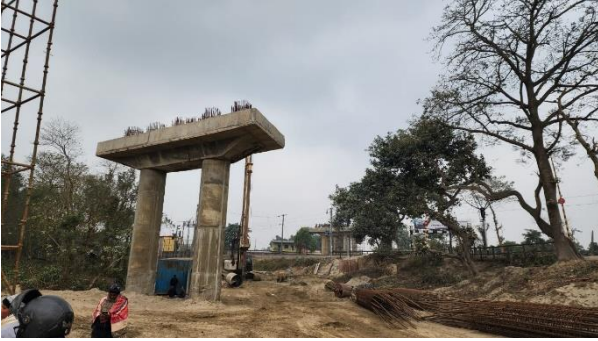
ROB Under Construction
